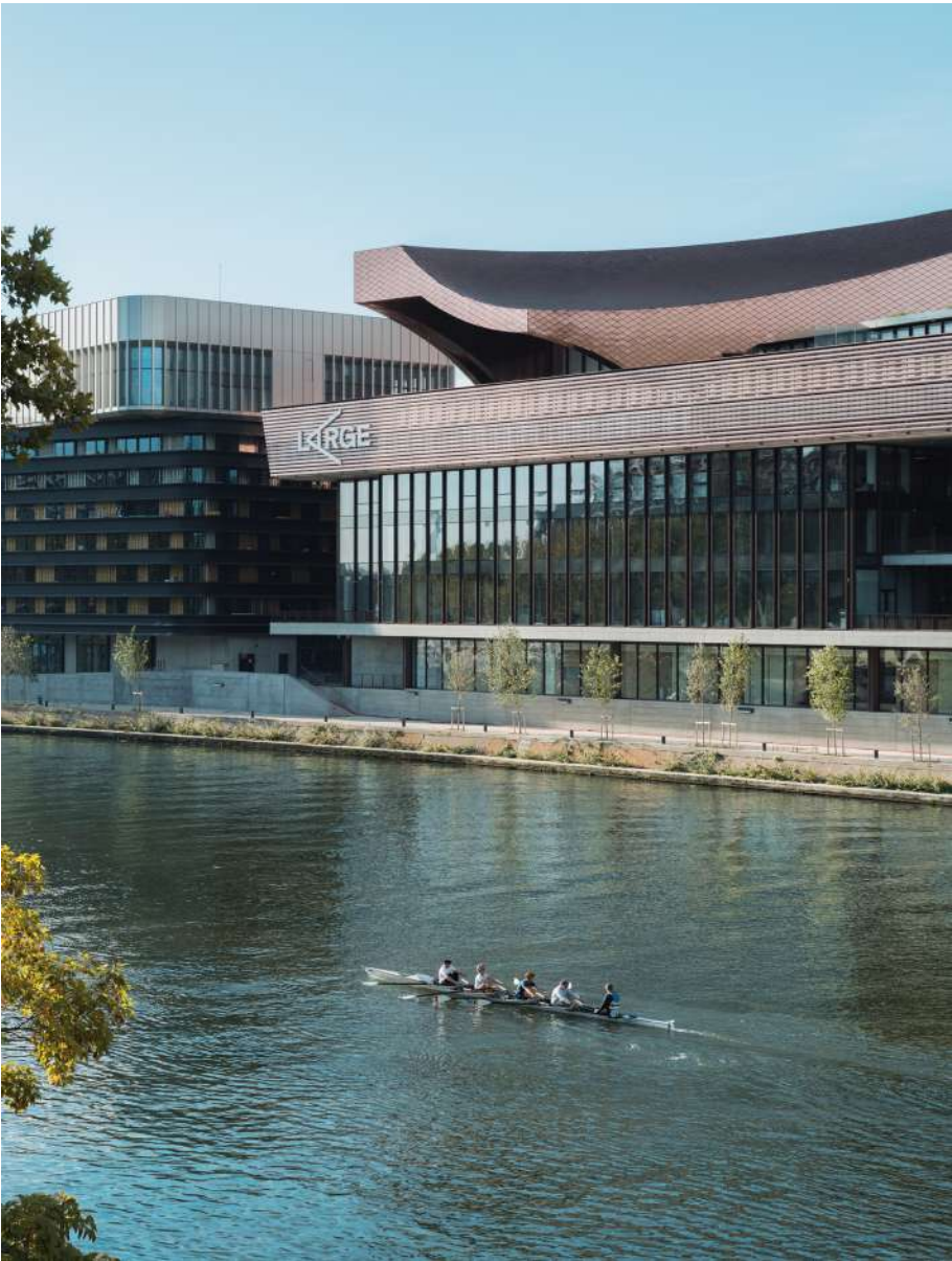
Large seen from the Seine, beneath the Seibert Bridge, Île Seguin, Boulogne-Billancourt, France. © RCR Architectes - G. Trégouët / CALQ agence d'architecture, Photographie © Nicolas Trouillard
